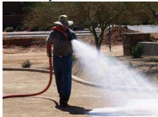
Standard Hose & Pump Hand Spraying
