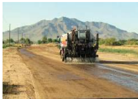
Unpaved Dirt Roads Unpaved Road Dust Control Gravel Road Dust Control Dirt Road Dust Control
