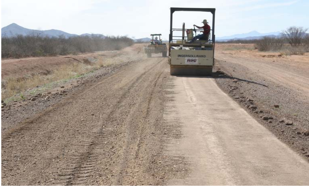
Figure 3. Compacting Soil after Mixing
