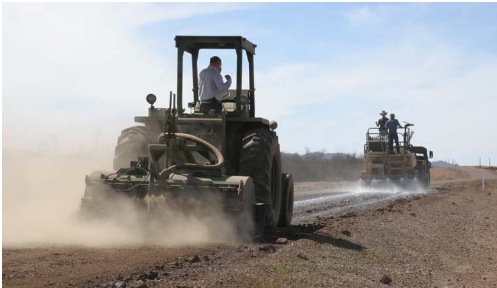
Figure 2. Applying Product with HydroSeeder and Mixing into Soil with Rotary Mixer
