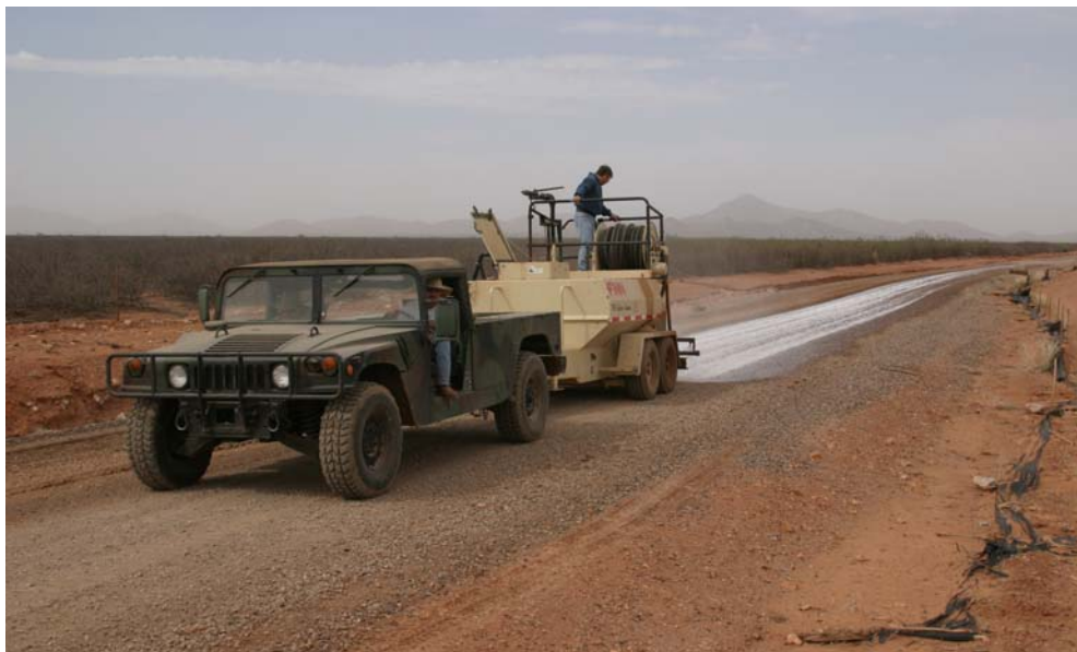
Figure 4. Applying Final Spray to Soil Surface after Compaction
