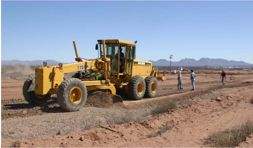
Figure 1. Grading Soil Surface before Treatment
