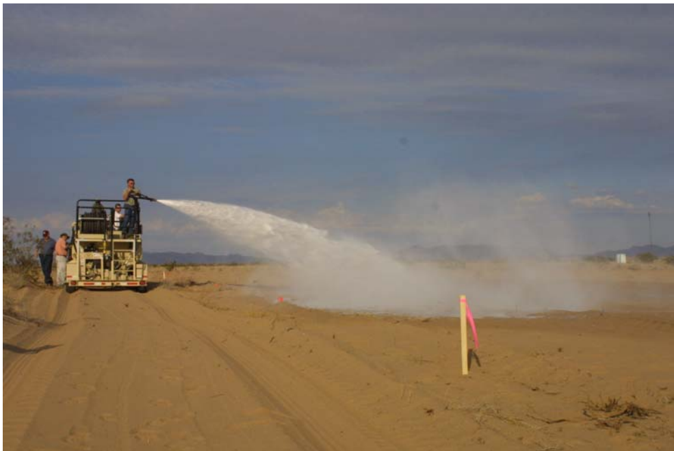
Figure 6. Topical Material Application from HydroSeeder Tower Gun
